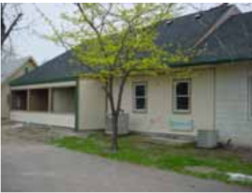
The windows are in and the screened porches are nearing completion.
