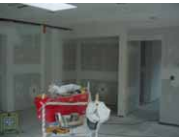
Hallmark employees generously donated their time to put up drywall.
